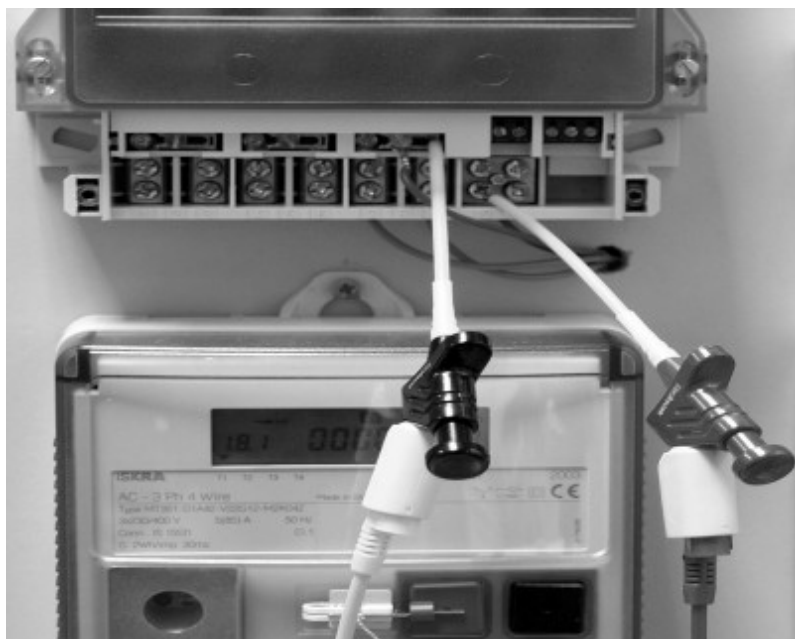
Connecting DLC SPY maintenance tool to the LV connection terminal of the meter unit
