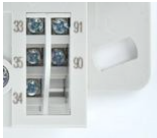
Figure 61: Service control terminal
